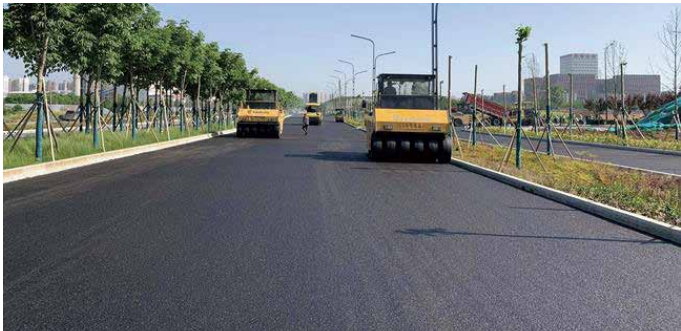
Municipal road pavement construction inspection and acceptance
