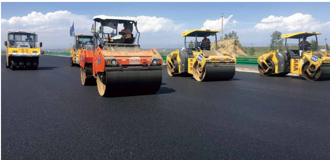
Highway pavement surface construction inspection and acceptance
