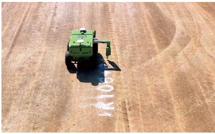
Pile Number Marking
