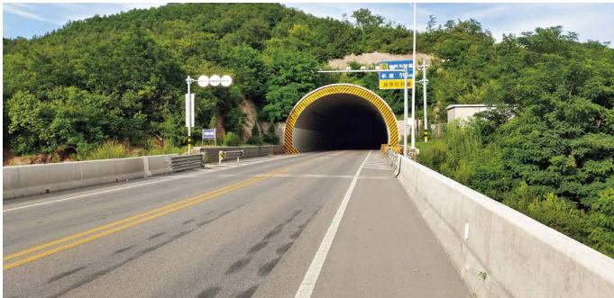
Regular inspection of key road sections, for proactive maintenance
